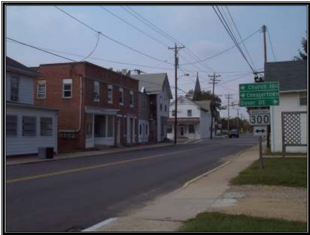
Approaching the intersection of MD 313 and MD 300. While these buildings are in need of maintenance and/or repair, they still represent a good example of commercial development in the Town Center in terms of scope, scale, and pedestrian orientation.
